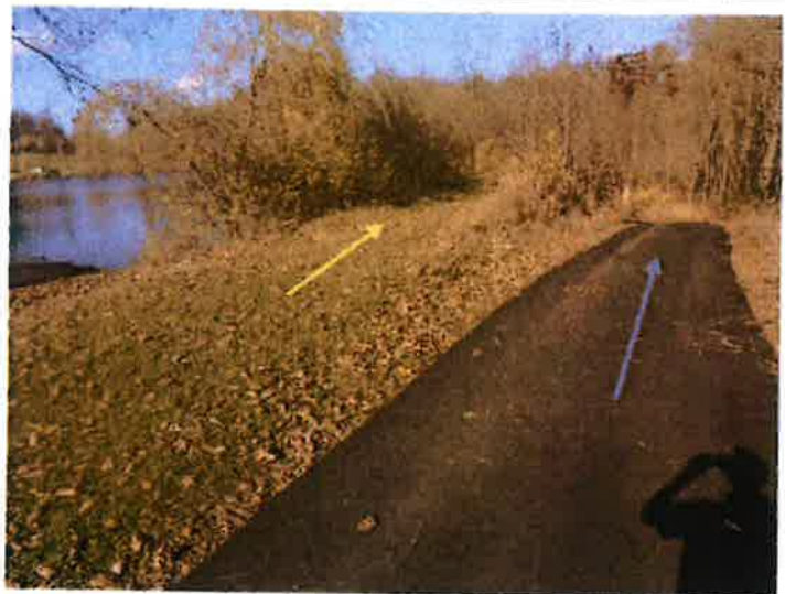
5. A view of the crest (yellow arrow) and downstream slope (blue arrow) from the right abutment.
