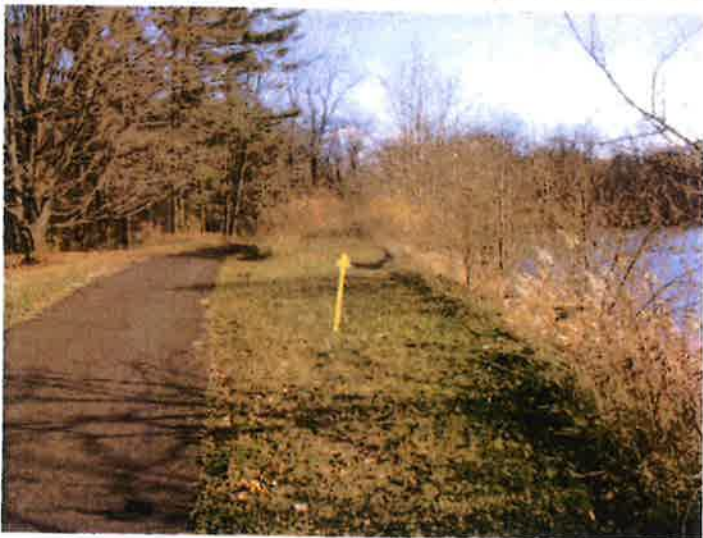
2. A view of the crest, upstream slope, and asphalt road leading down the downstream slope. The 10-foot-wide crest is indicated by the yellow arrow. This view is from the left abutment.
