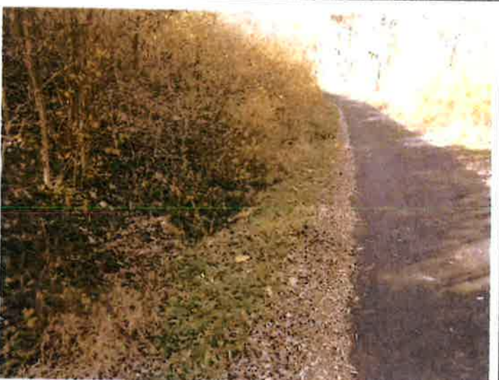
6. A view of the downstream slope looking left. Note that the dense trees and brush prevented a thorough investigation of the slope.
